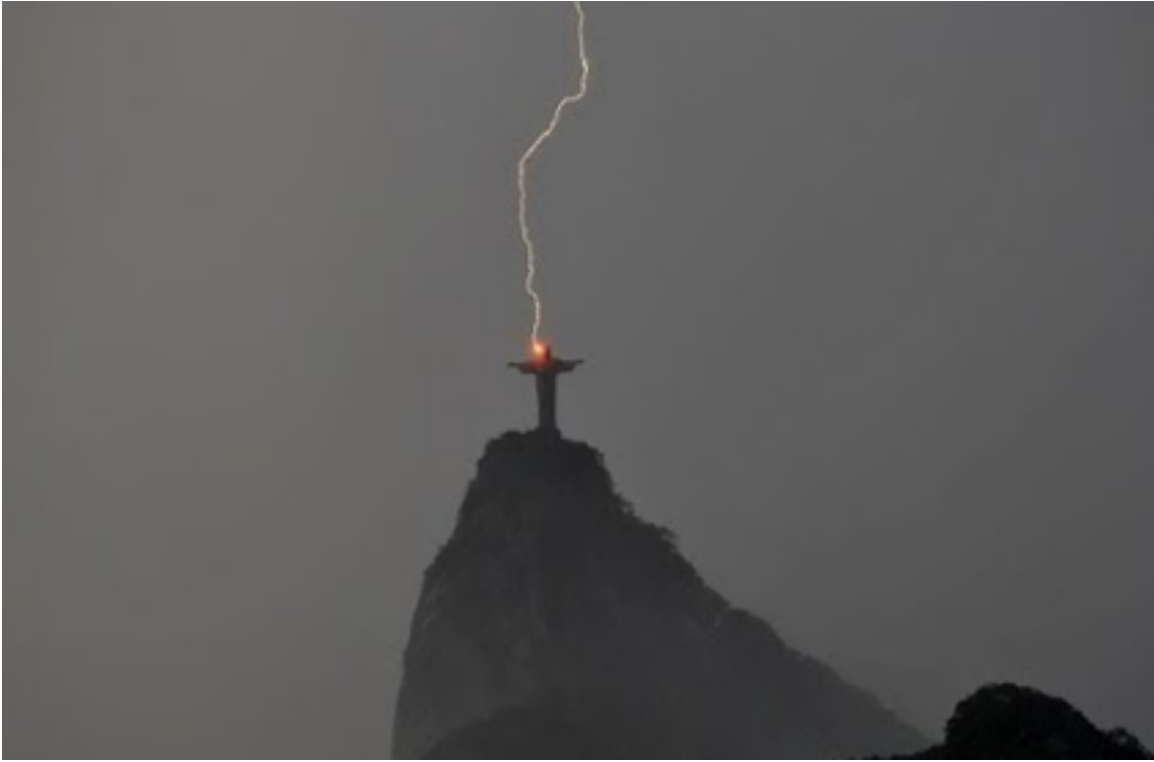
Lightning strikes the statue of Christ in Rio de Janeiro, Brazil, during a storm in 2014, chipping the right thumb.
